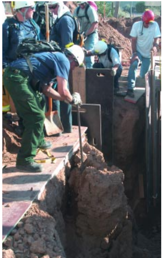
In this photo, an instructor supervises a student knocking down an unstable column of soil prior to beginning shoring operations. The instructor must define the acceptable risks and make the operation safe.
